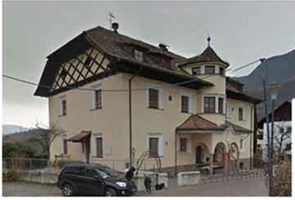
Elementary School – Missiano BZ (Italy) 2 x POWER HT + 110
